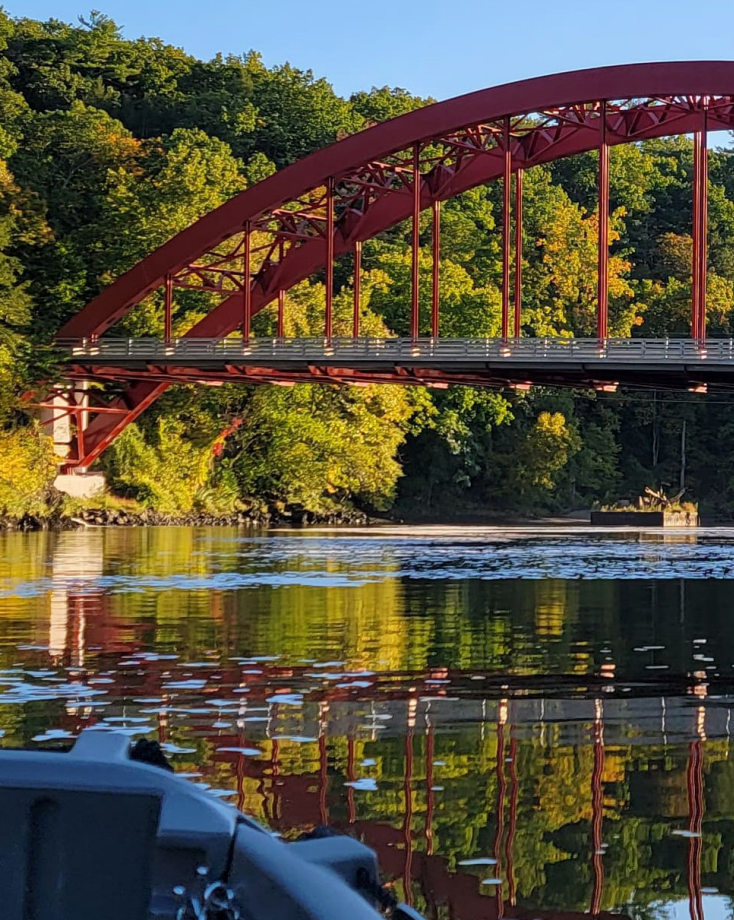
Image: The Eddyville Bridge over Rondout Creek in Ulster County, New York.
